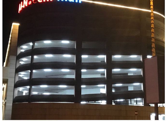
AI-Naeem Mall-RAK LED Parking & Retrofit Lighting
