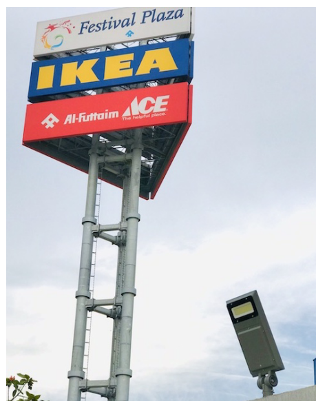
Festival Plaza Solar Street Lighting
