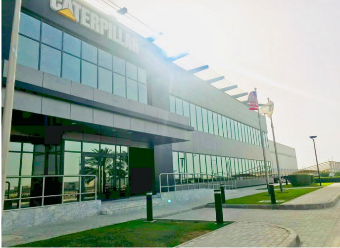
Caterpillar-Dubai LED & Solar Landscape Lighting
